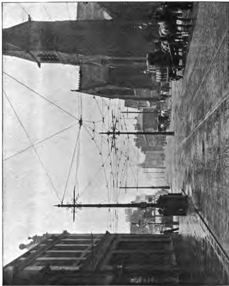
FIG. 16. CROSS LANE JUNCTION, SALFORD. THE LARGEST AND MOST COMPLICATED OVERHEAD TROLLEY CROSSING IN THE KINGDOM
